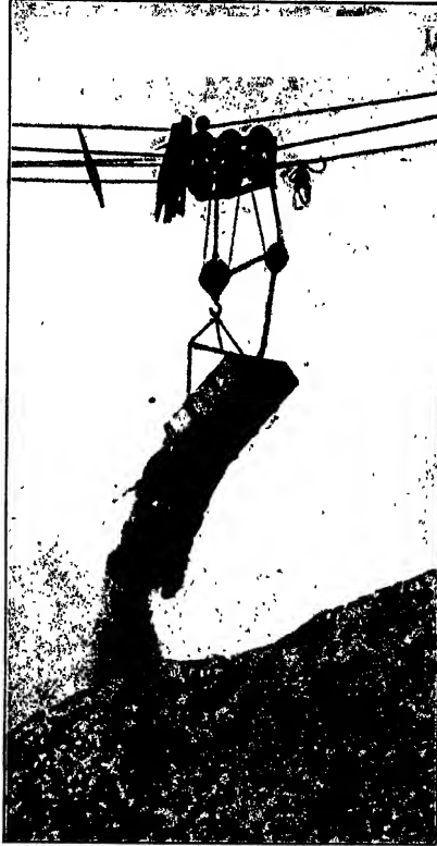
FIG. 139.—Installation for Hoisting and Conveying : Aerial Dump.
